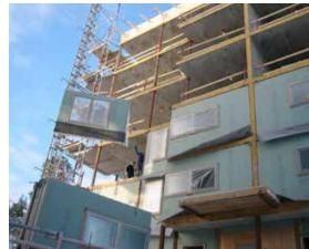
Wood infill walls in a concrete frame.
