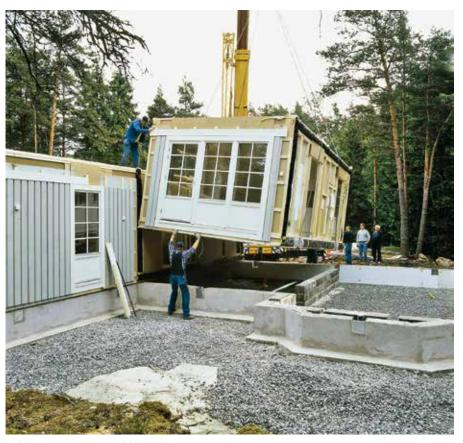
Volumetric units are assembled on the construction site.
