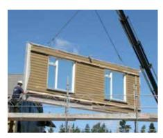
A surface unit is delivered to the construction site.
