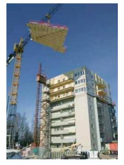
Three additional storeys in wood added to an existing concrete building.
