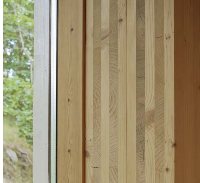
External wall made of CLT.
