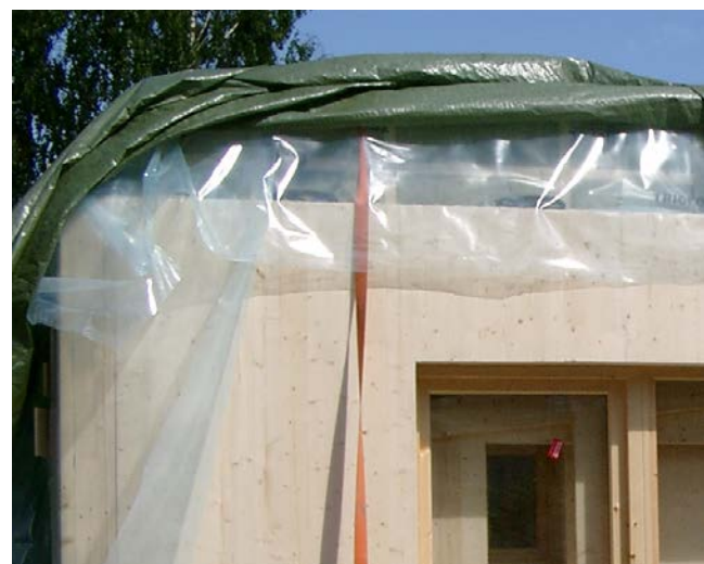
Prefabricated wall elements being unwrapped.
