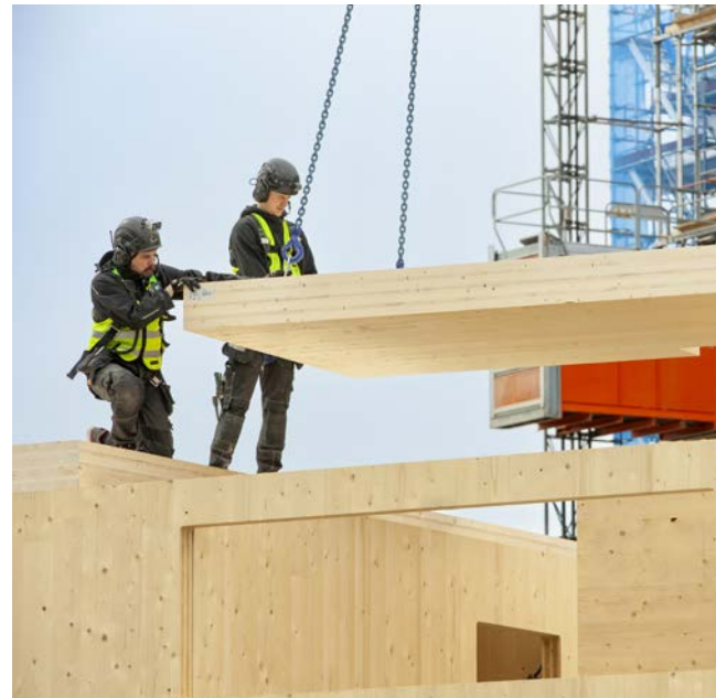
Installing a CLT floor slab.
