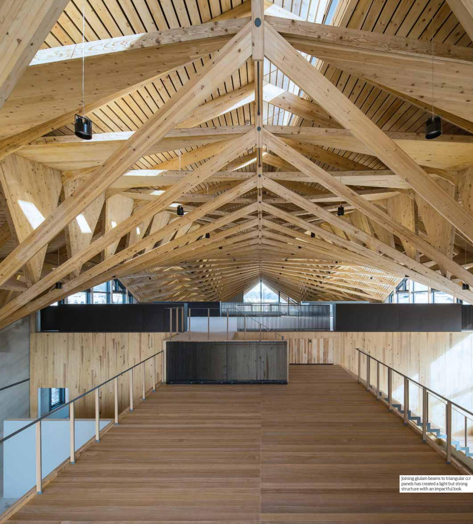
Joining glulam beams to triangular CLT panels has created a light but strong structure with an impactful look.
