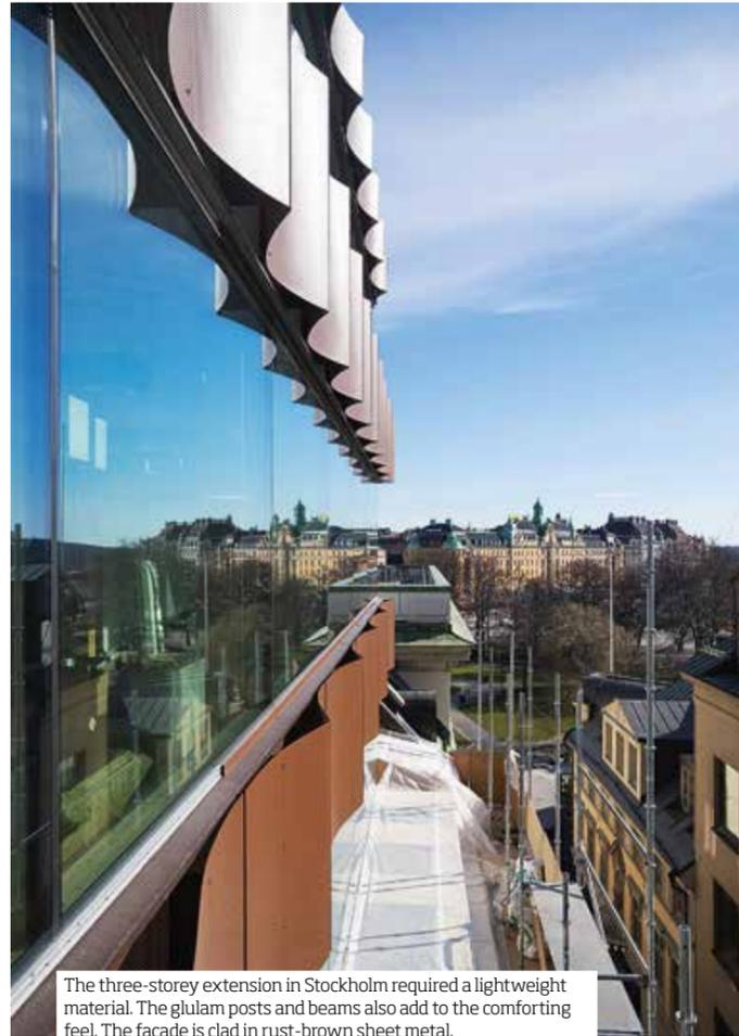
The three-storey extension in Stockholm required a lightweight material. The glulam posts and beams also add to the comforting feel. The façade is clad in rust-brown sheet metal.
