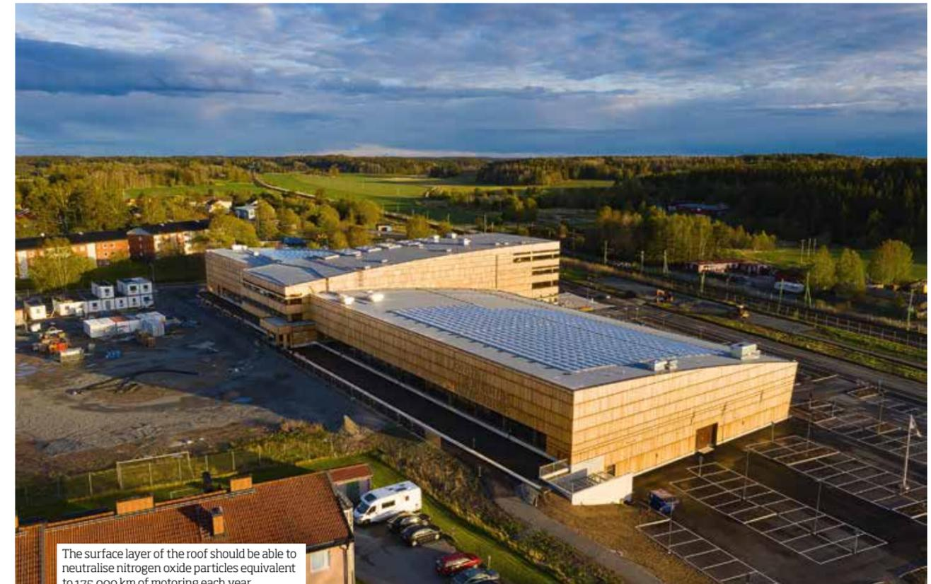
The surface layer of the roof should be able to neutralise nitrogen oxide particles equivalent to 175,000 km of motorway each year.
