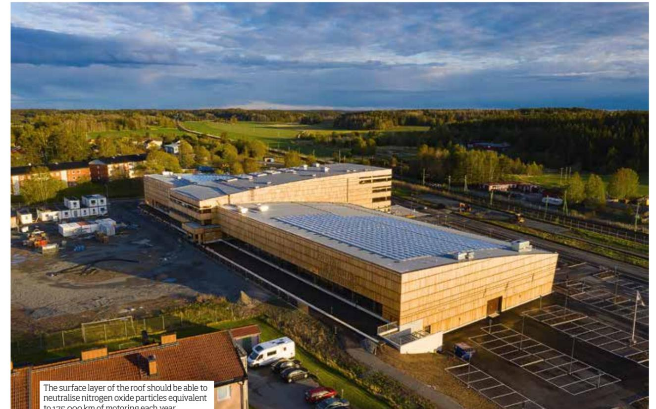
The surface layer of the roof should be able to neutralise nitrogen oxide particles equivalent to 175,000 km of motoring each year.
