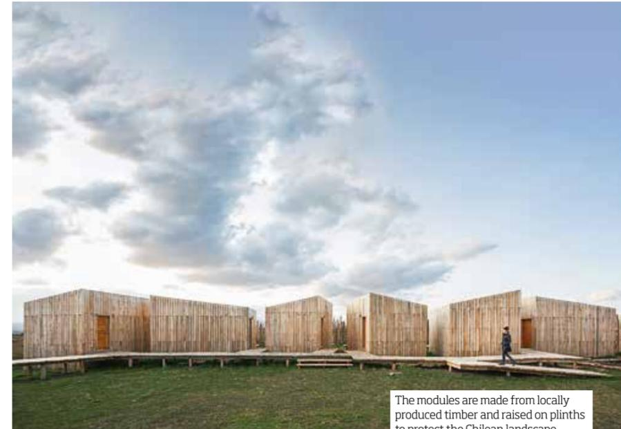
The modules are made from locally produced timber and raised on plinths to protect the Chilean landscape.
