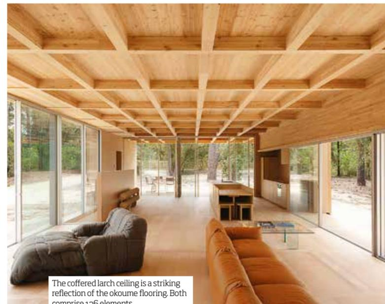
The coffered larch ceiling is a striking reflection of the okoume flooring. Both comprise 136 elements.
