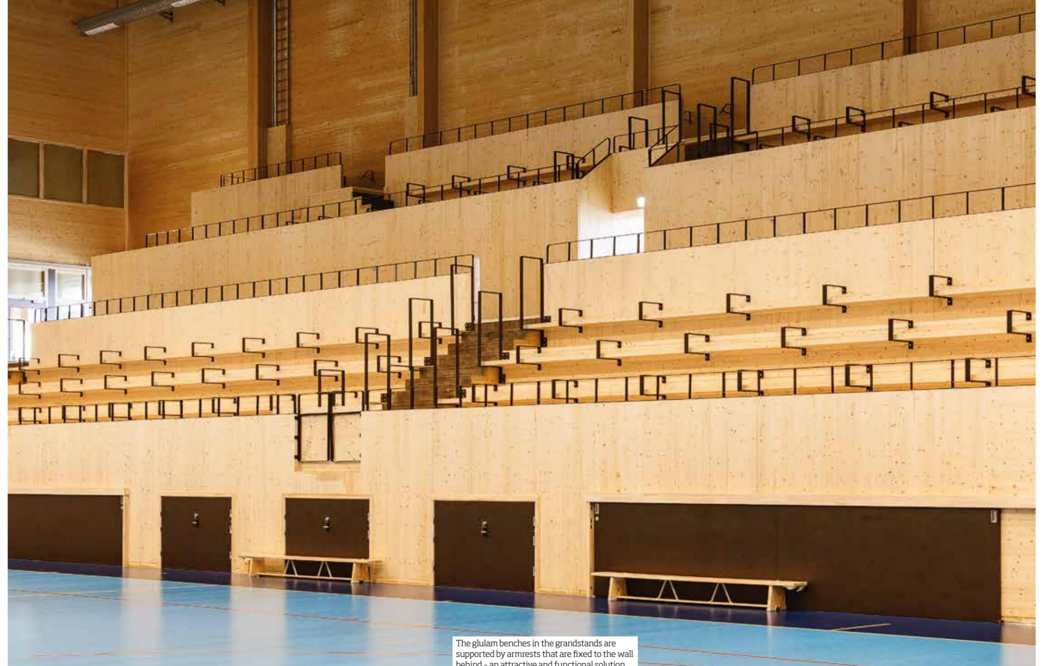
The glulam benches in the grandstands are supported by armrests that are fixed to the wall behind – an attractive and functional solution.
