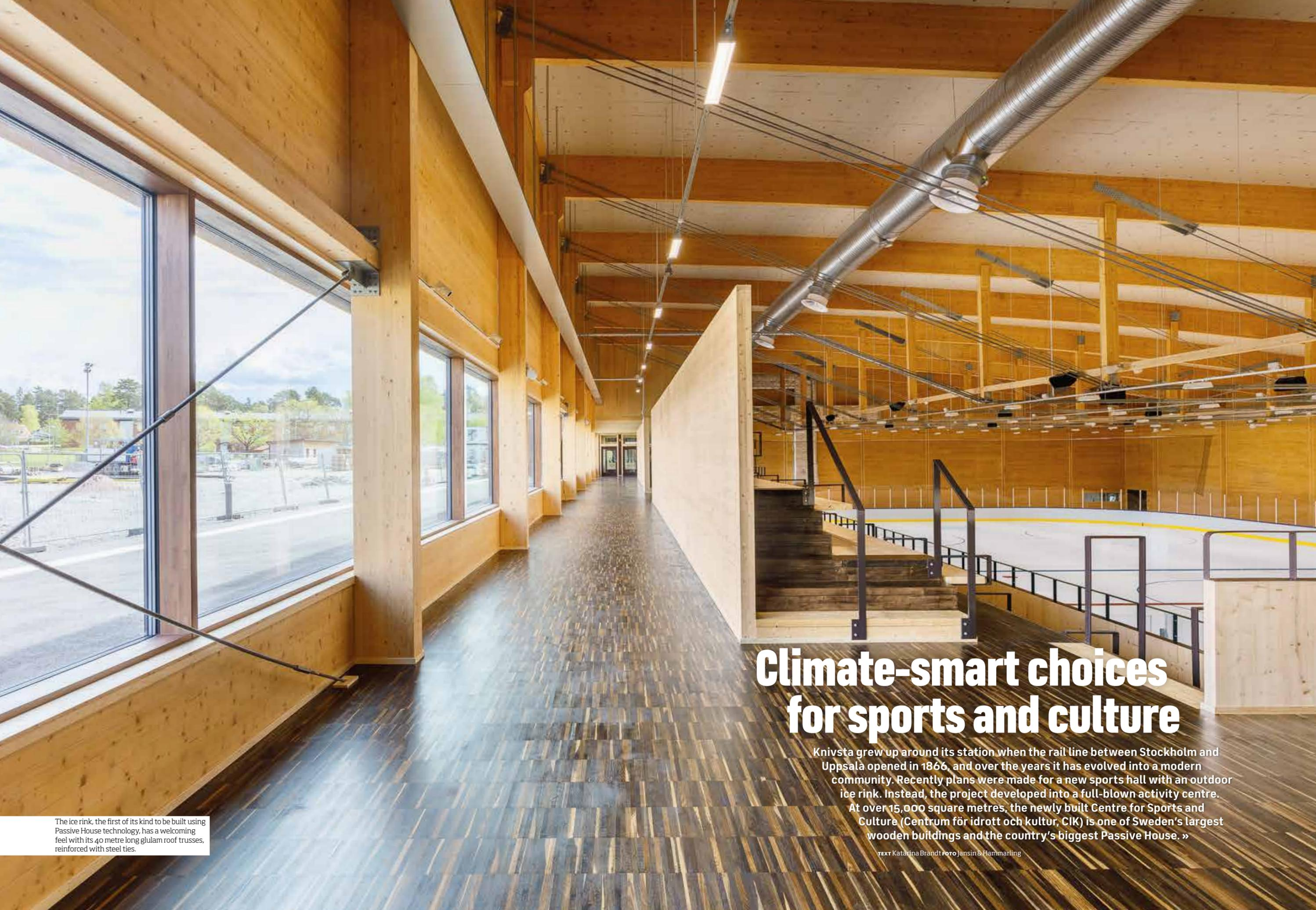
The ice rink, the first of its kind to be built using Passive House technology, has a welcoming feel with its 40 metre long glulam roof trusses, reinforced with steel ties.
