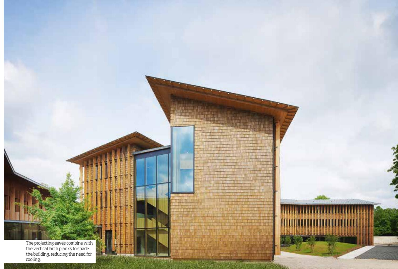
The projecting eaves combine with the vertical larch planks to shade the building, reducing the need for cooling.
