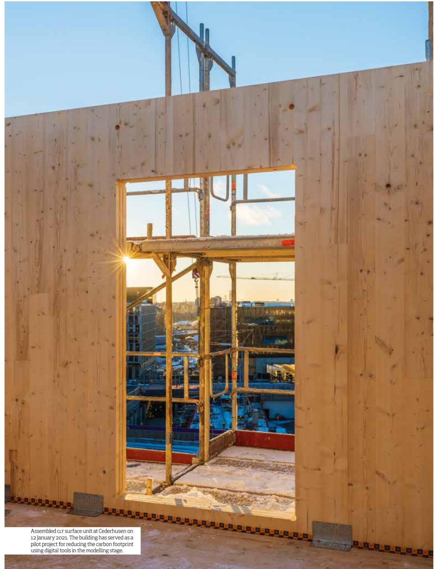
Assembled CLT surface unit at Cederhusen on 12 January 2021. The building has served as a pilot project for reducing the carbon footprint using digital tools in the modelling stage.
