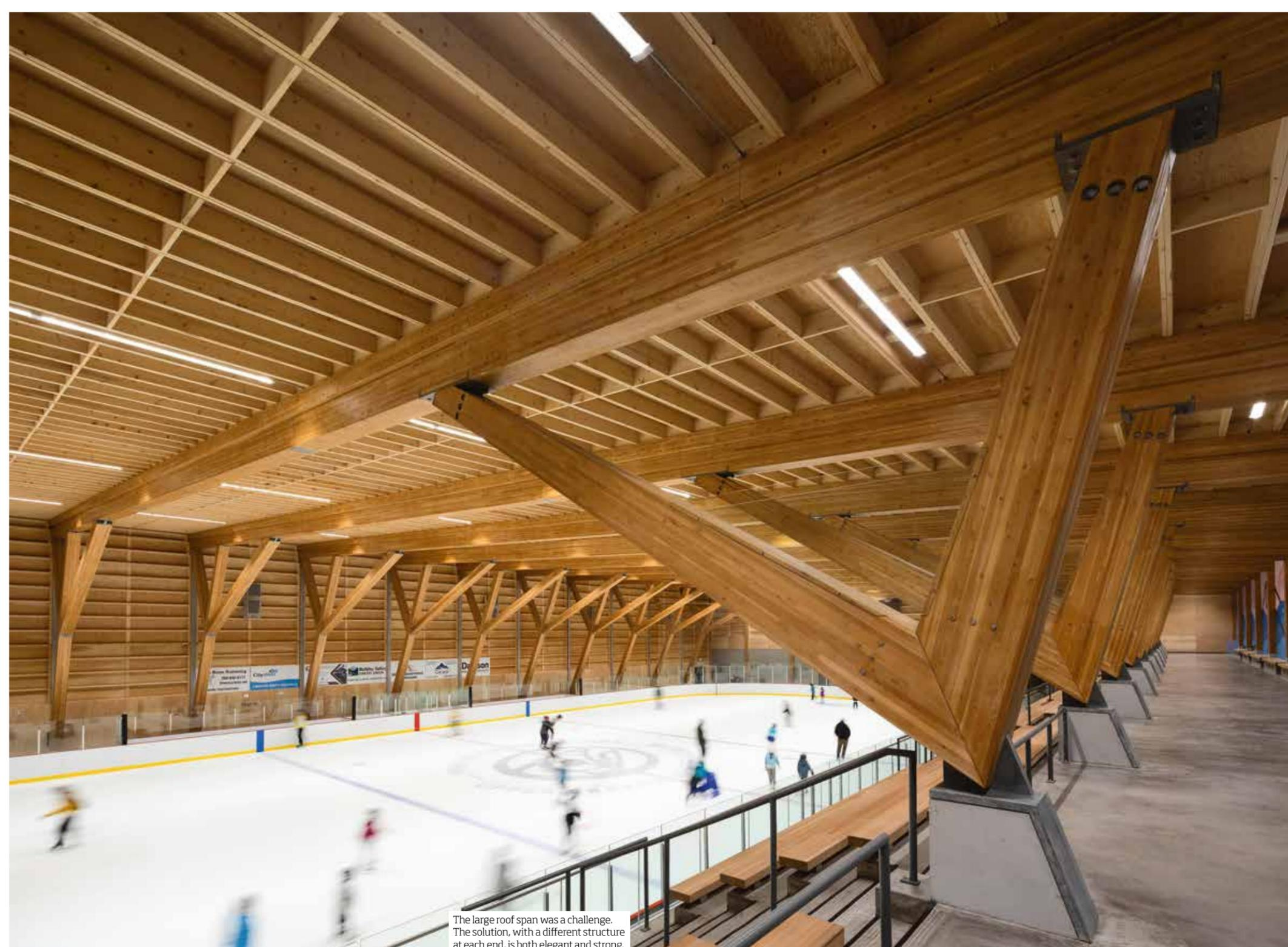
The large roof span was a challenge. The solution, with a different structure at each end, is both elegant and strong.
