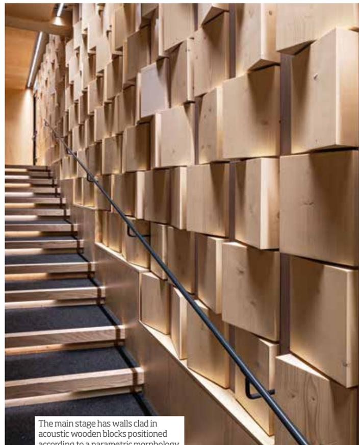
The main stage has walls clad in acoustic wooden blocks positioned according to a parametric morphology.
