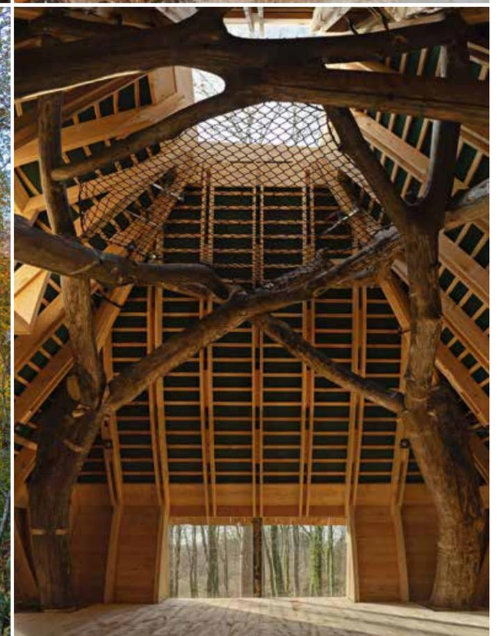
The strength is optimal in the tree forks, and the students at Hooke Park are exploring how they can be put to structural use.
