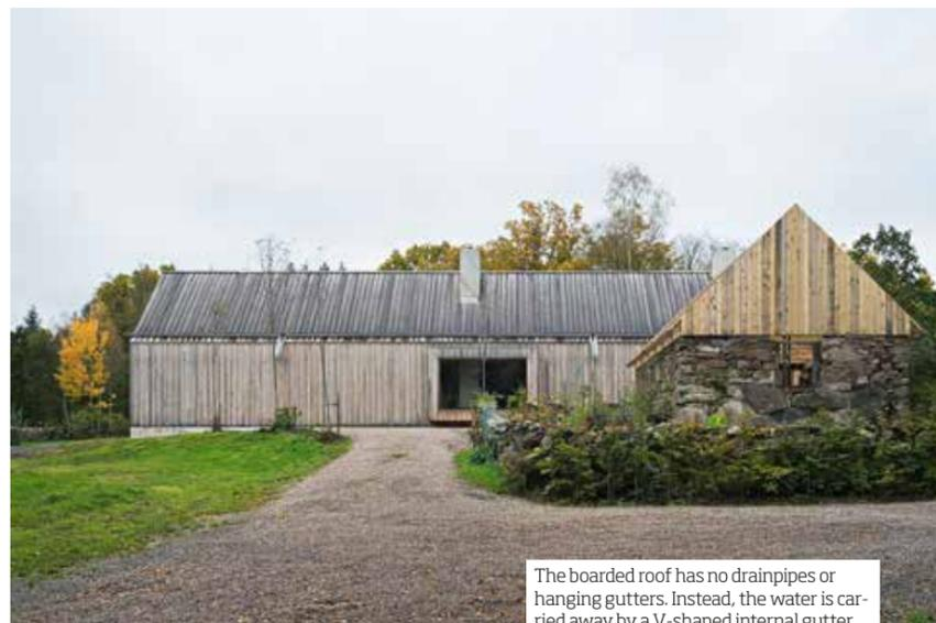
The boarded roof has no drainpipes or hanging gutters. Instead, the water is carried away by a V-shaped internal gutter.
