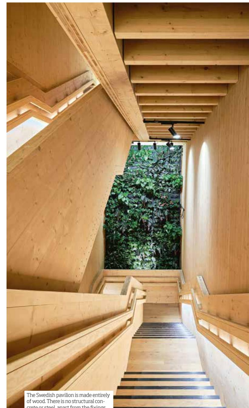
The Swedish pavilion is made entirely of wood. There is no structural concrete or steel, apart from the fixings.
