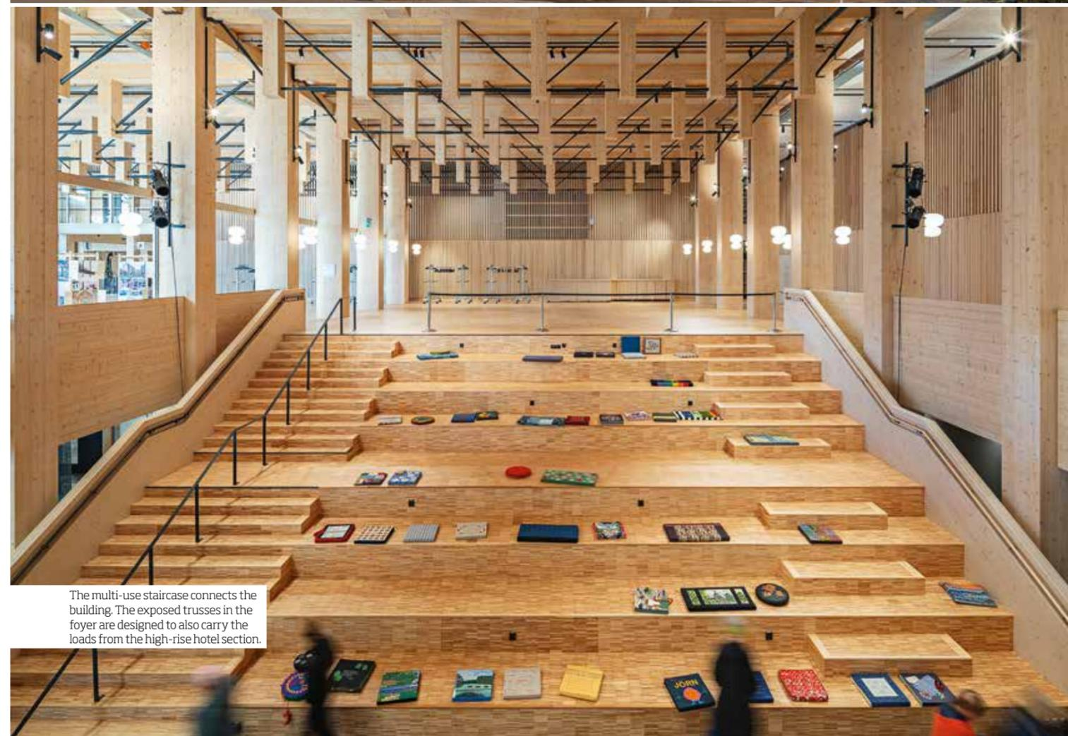
The multi-use staircase connects the building. The exposed trusses in the foyer are designed to also carry the loads from the high-rise hotel section.
