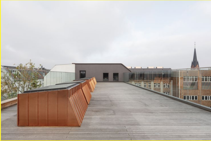
Externally, the extension's copper cladding matches the warm tones of the original brick-slip facade, while at the same time distinguishing the new intervention from the existing building.
