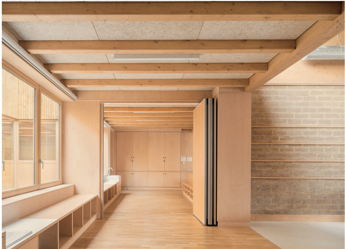
The building has, alongside the load-bearing masonry walls, a load-bearing frame of CLT and glulam as well as interior walls of compressed air-dried clay brick.
