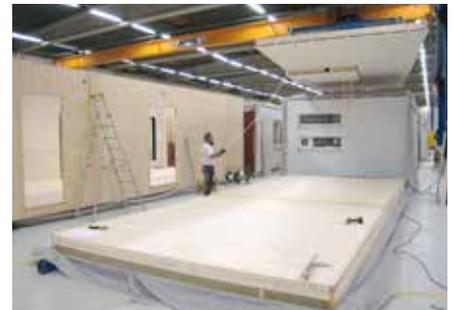
*Prefabrication of volumetric units.*
