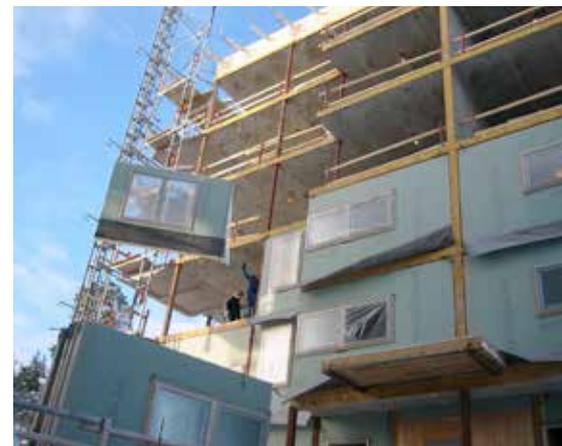
Wood infill walls in a concrete frame.
